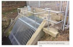
Screens must be installed at certain interval on the surface drains to arrest the solid waste from moving ahead and clogging the drain. The solid waste shall be raked regularly depending upon the screenings collected. The community must be sensitized regarding hazards of disposal of solid waste in the drains. The drain shall also be cleaned regularly to remove the grit and unwanted vegetation if any. These tasks are to be performed using mechanical instruments shown on the subsequent slides.
