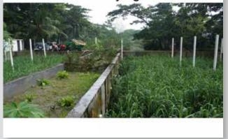
A planted drying bed is a type of drying bed which uses plants (macrophytes) to stabilize and dewater the sludge.
