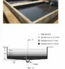
Sludge drying beds are mainly used for dewatering of stabilized sludge.
