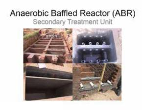
Left up: Two street ABR under construction Right up: Baffled pipes Right down: Fixing of outlet pipes Left down: First chamber with baffled wall instead of pipes for better flow distribution.
