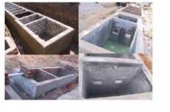
Left up: Integrated settler + anaerobic baffle reactor Right up: Openings in settler divider wall Right down: Openings and gas vent pipe in divider wall Left down: Connection of inflow and outflow pipes (without T-pipe at this stage)
