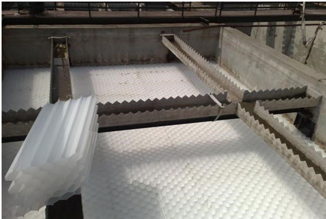
Figure 50: Example of tube settler media for retrofitting secondary clarifier
