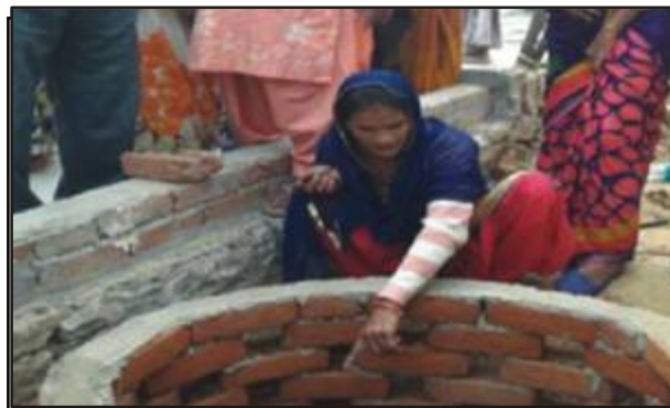
CMC women explaining the Twin Pit Technique at Jawahar Nagar as part of SAHAY Single Widow Initiative
