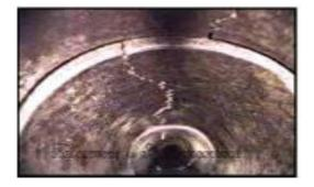
Photographs showing Structural Damage and Longitudinal cracked condition of the Sewer
