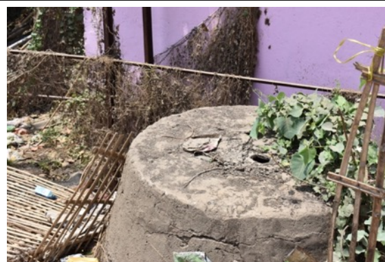
Decanting point outside the STP
