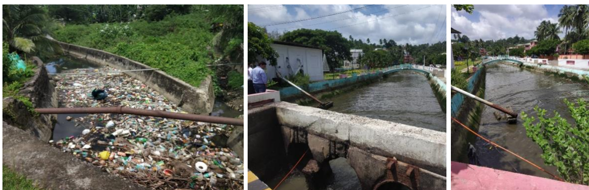
FIGURE 11: A) THE BIGGER STORM WATER DRAINS WITH SOLID WASTE B) BIGGER STORM WATER DRAIN NEAR CITY GARDEN
