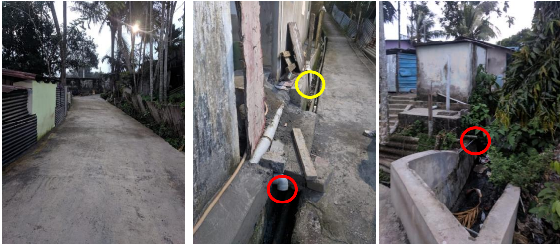
FIGURE 10: A) STORM WATER DRAIN COVERED WITH CONCRETE ROAD B) & C) DISCHARGE OF GREY WATER AND BLACK WATER DIRECTLY INTO THE STORM WATER DRAINS
