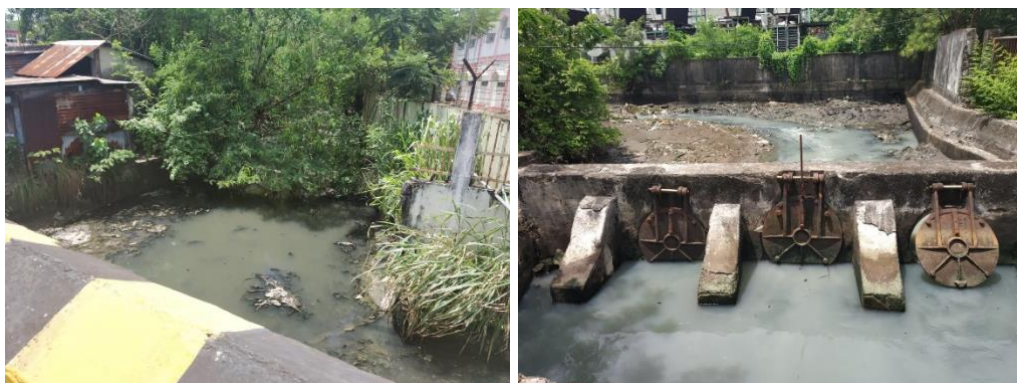
FIGURE 7: A) BIGGER STORM WATER DRAIN WHICH HAS WASTEWATER DISCHARGE B) OUTFALL IN THE SEA NEAR FISHERIES JETTY
