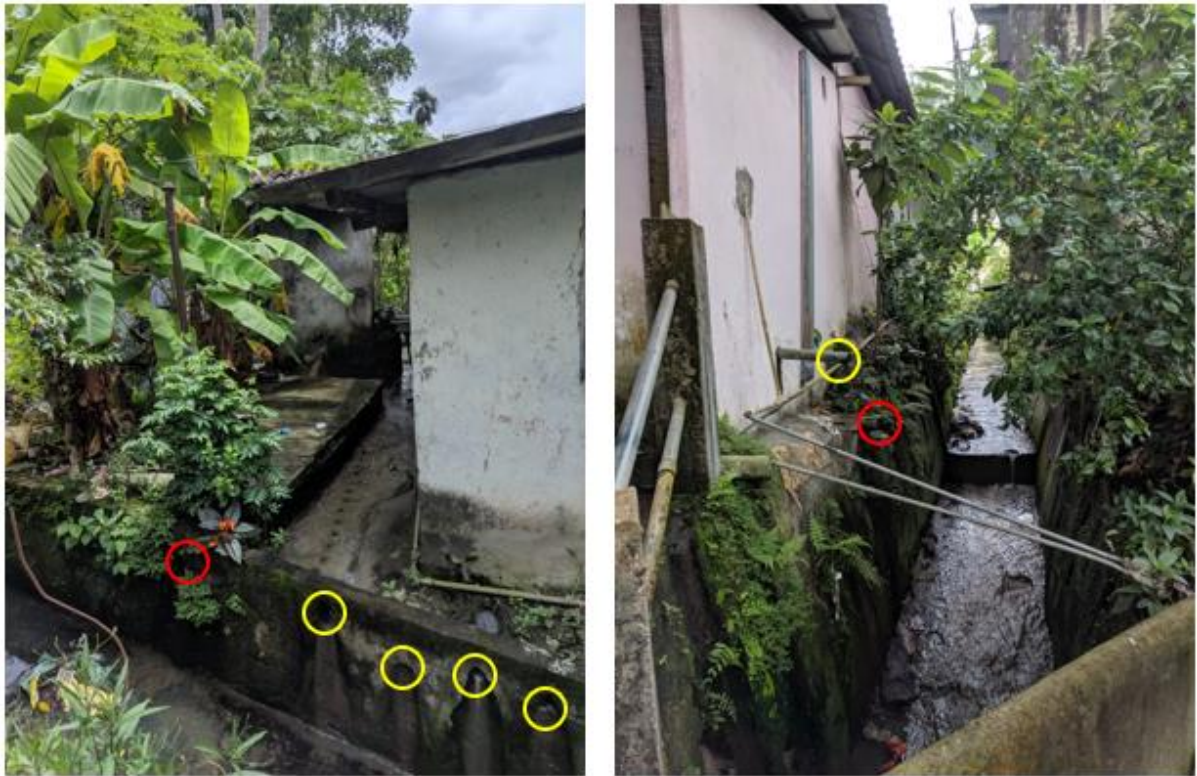
FIGURE 3: DISCHARGE OF SEPTIC TANK AND GREY WATER FROM HOUSEHOLDS INTO THE STORM WATER DRAIN OBSERVED AT POINT A (RED CIRCLES SHOWS THE SEPTIC TANK OUTLET AND YELLOW CIRCLE DENOTES GREY WATER OUTLET)
