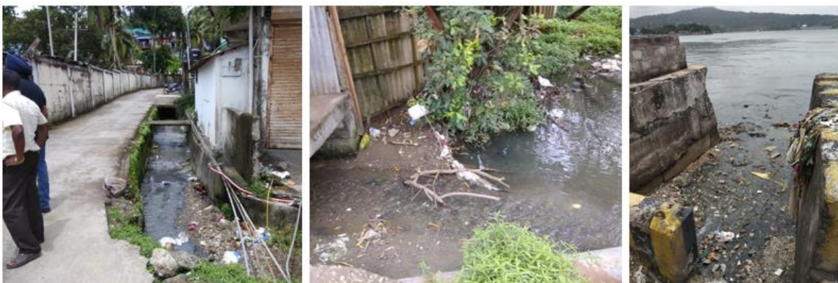
FIGURE 4: (A) CONCRETE ROAD AT POINT B (B) SOLID WASTE DUMPED IN THE DRAINS AT POINT A (C) OUTFALL OF THE STORMWATER DRAINS IN TO THE SEA AT POINT B
