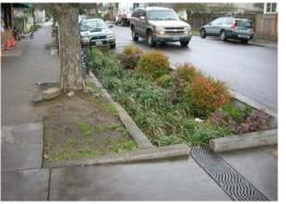
Figure 16 Roadside swales installation
