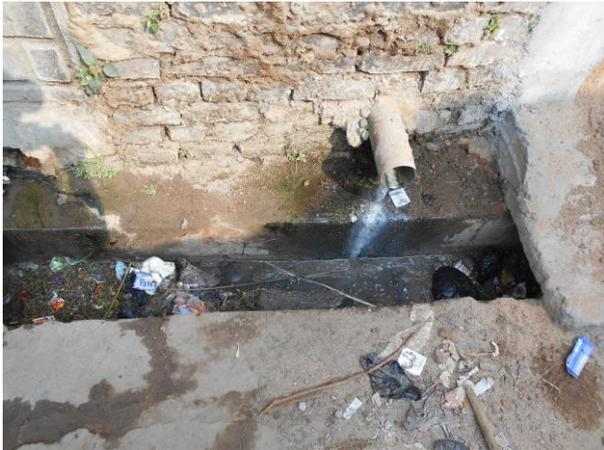
**Figure 9: Outlet of a containment unit drains directly into a drain**
