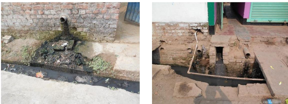
Figure 1: Outlet of Containment Units overflowing into drains
