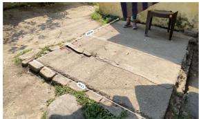
Figure 3 Lined tank with impermeable wall and open bottom (Source: Sachin Sahani/NIUA/2021)
