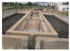
Figure 19 Twin settling-thickening tanks of Rufi sque faecal sludge management plant, in Dakar, Senegal (Source: SANDEC)
