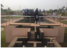
*Figure 18 Settling thickening tank, Bhubaneshwar (Source: Dhawal Patil, ESF)*
