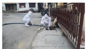
Figure 6 Emptying of Septic tank connected to open drain (Source: Jheelam Sarkar/NIUA/2022)
