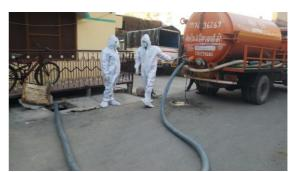
Figure 7 Spillage of Septage during Desludging (Source: Jheelam Sarkar/NIUA/2022)
