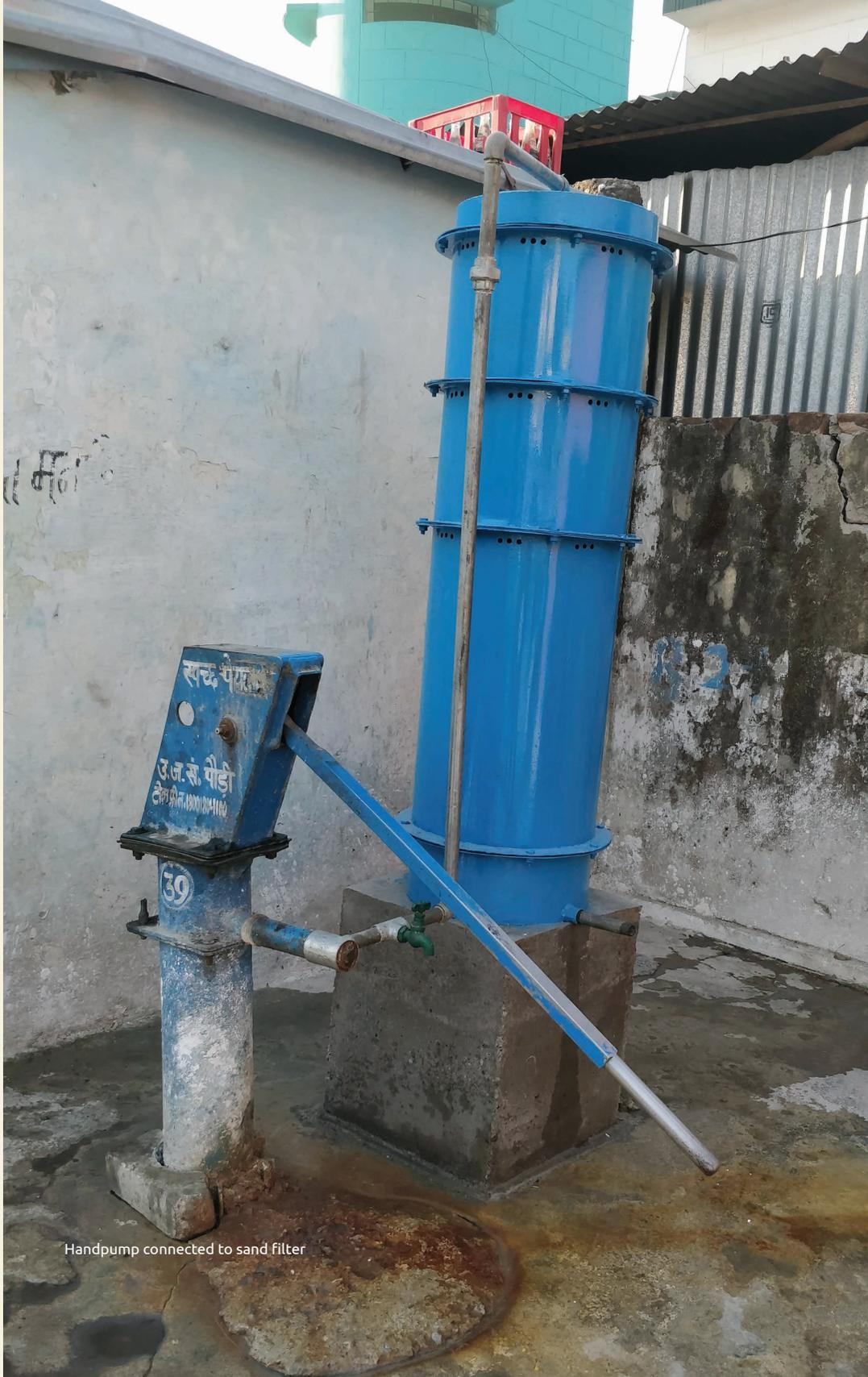
Handpump connected to sand filter
