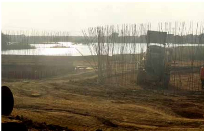
Figure 5: STP work in progress at Chintal cheruvu Tank
