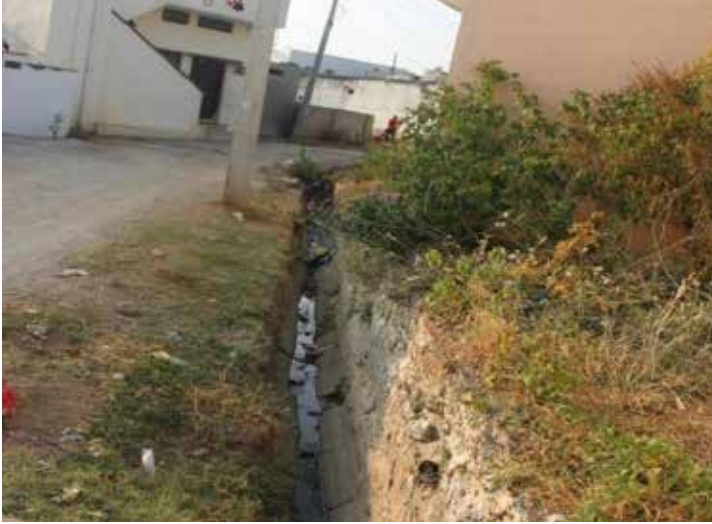
Figure 21: Old Drains with V shaped slope with shabad stone
