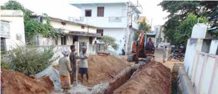
Figure 8: UGD work in progress
