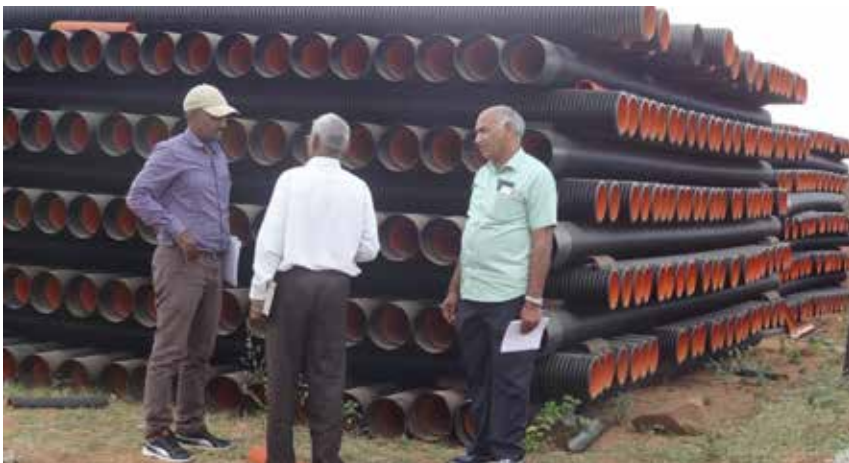
Figure 9: Pipelines used for developing UGD network
