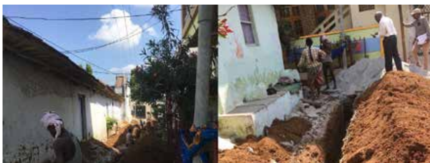
Figure7: UGD Pipeline work with manual labour
