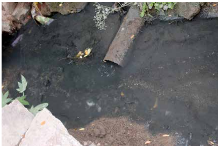
Figure 33: Household toilet outlet into the sewer drain
