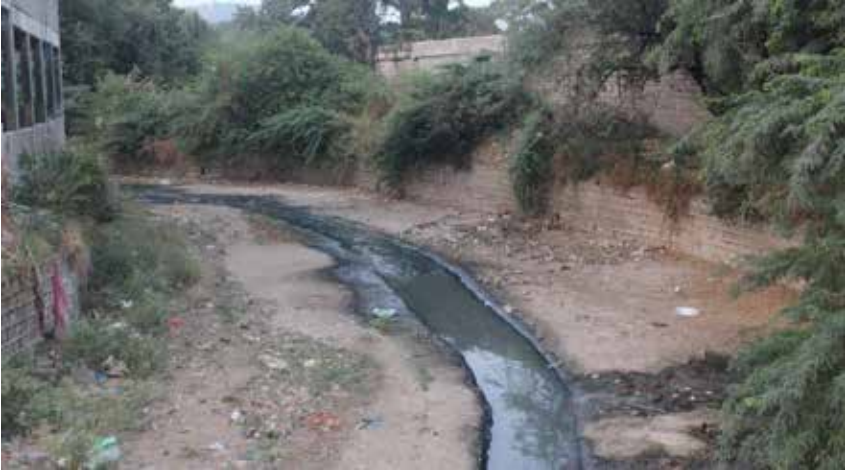
Figure 20: Storm water drain filled with silt
