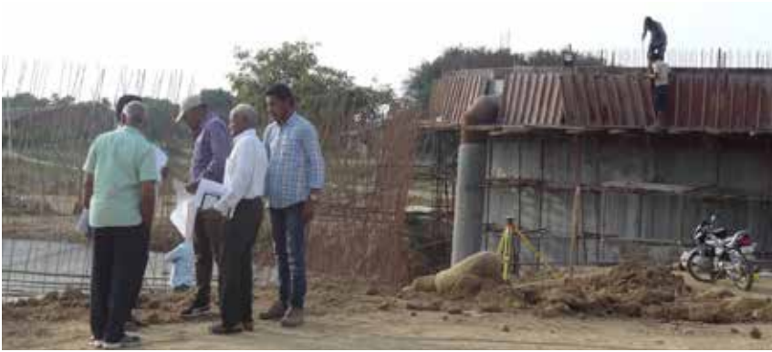
Figure 6: STP work in progress at Chintal cheruvu Tank
