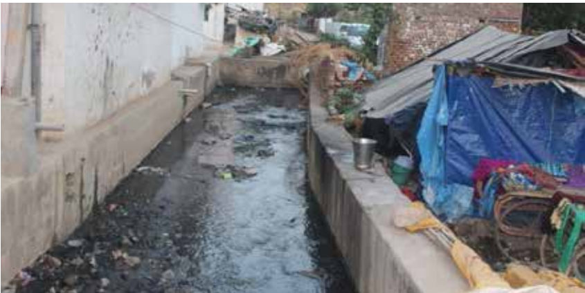
Figure 20: Storm water drain filled with silt
