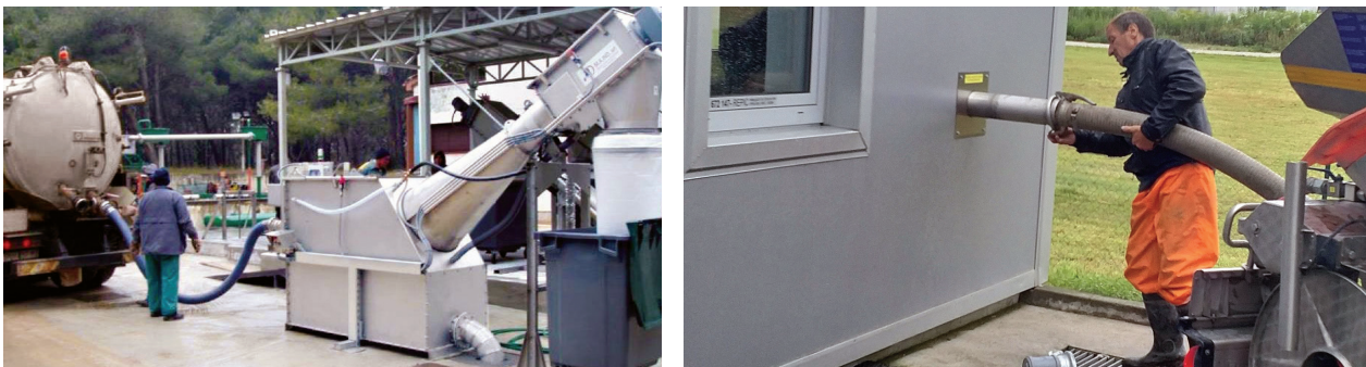
Figure 64: Typical photographs of the septage receiving station
