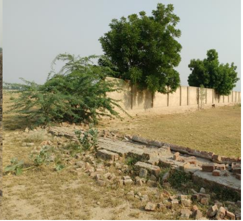
Figure 25: Existing compound wall at site
