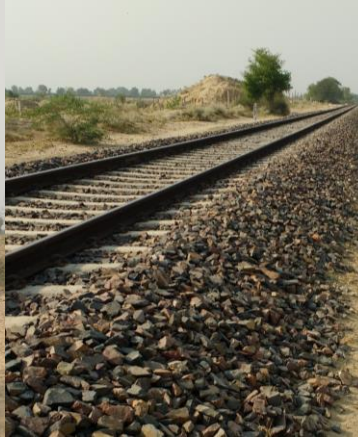
Figure 24: Railway track on westside of site
