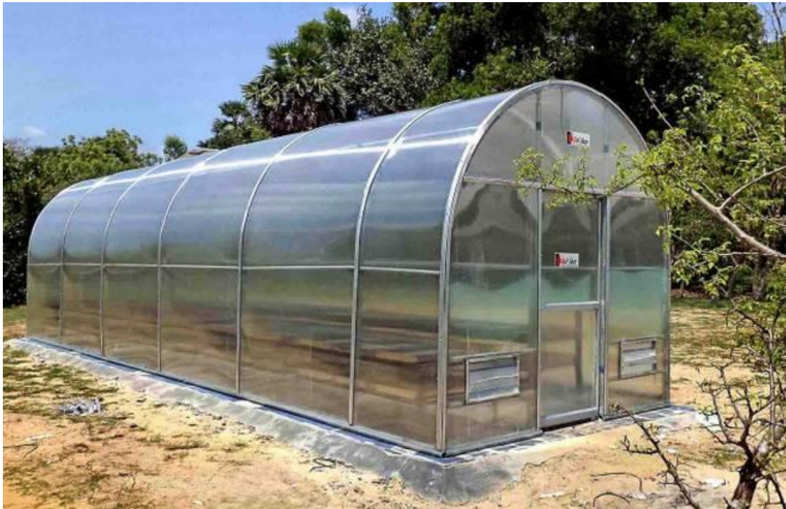
Figure 30: Sludge Sterilisation Unit
