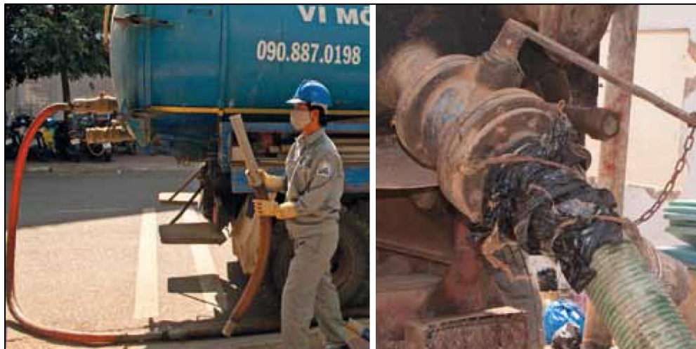
Figure 42: Correct and incorrect desludging method
