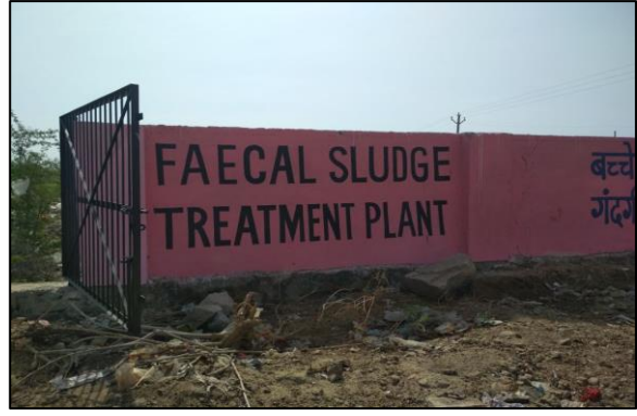
Figure 45: Existing compound wall at site
