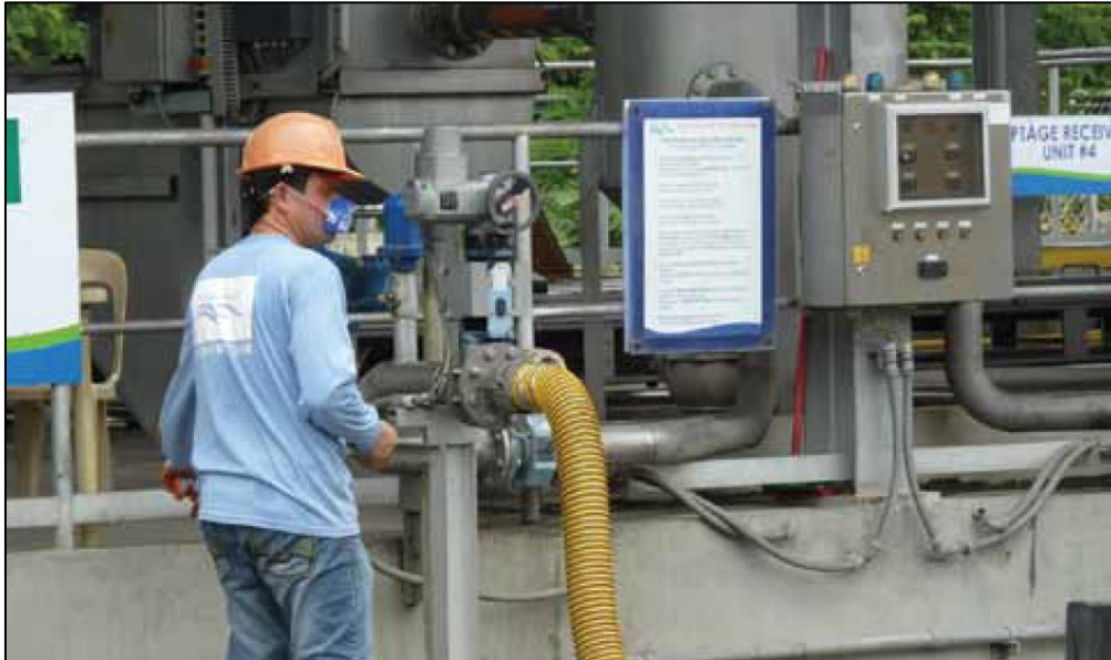
Figure 43: Unloading of tank
