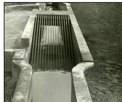
Figure 25: Screening chamber
