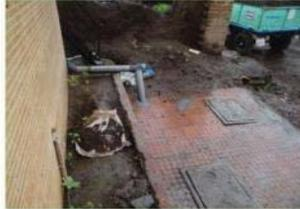
Toilets directly connected to drains
