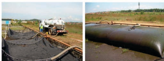
Figure 46: Geo-tube before and after use in Malaysia
