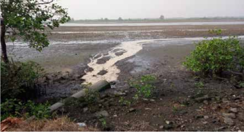
Figure 16-17: Sewerage from the private drains is discharged into the river at low tide and is carried to the sea during high tide
