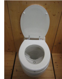
Urine Diversion Flush Toilet Western Two Hole Pan
