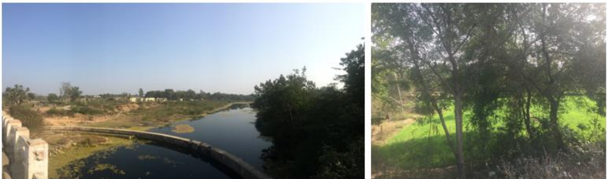
FIGURE 21: LOCATION OF THE STP (PICTURE 2) NEAR THE DO NADI BRIDGE (PICTURE 1) IN DUNGARPUR CITY
