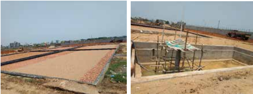
Figure 2.4 Pictures of Bhubaneswar FSTP
