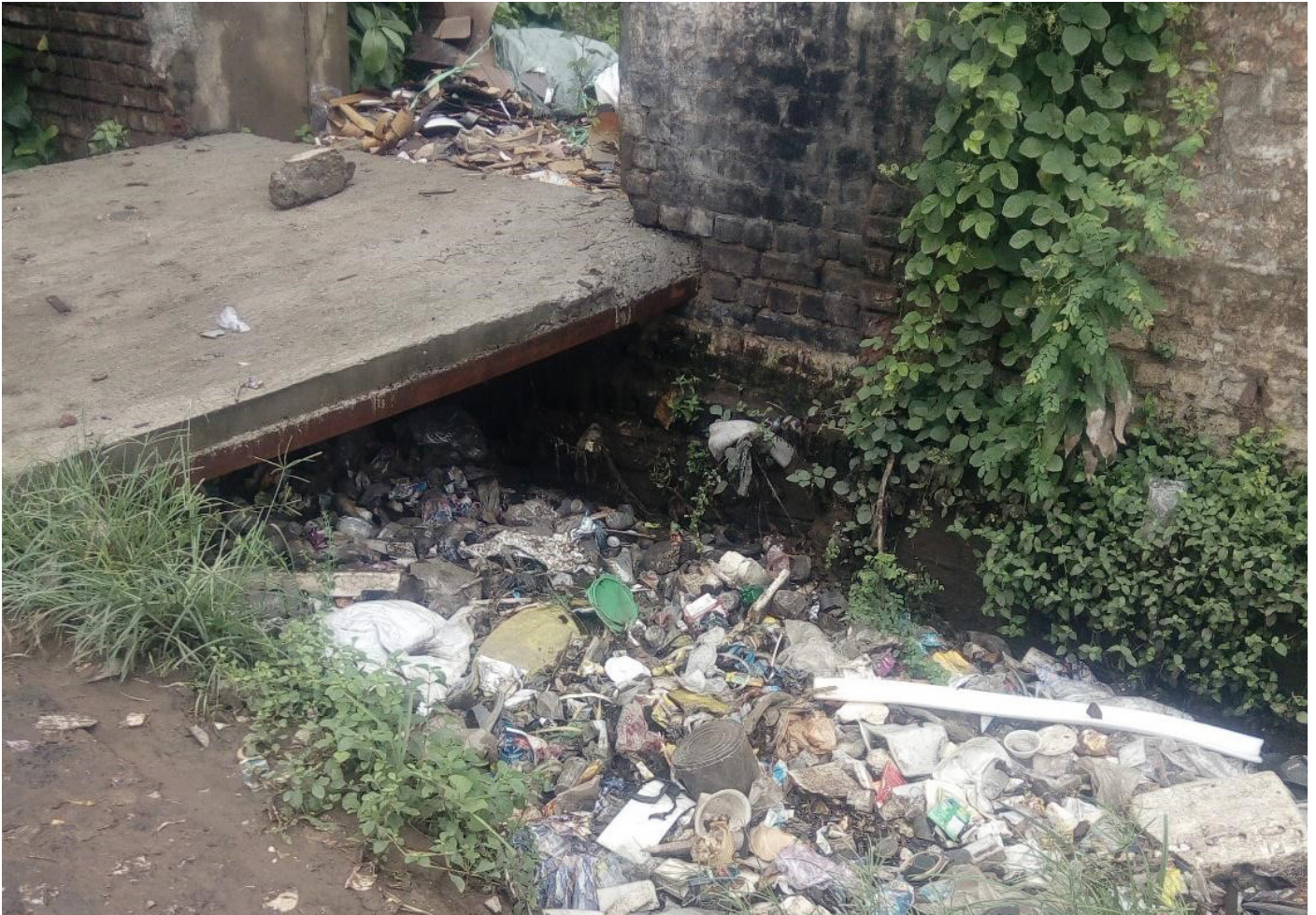
Fig. 13: Open Drain in Telibandha Area of Raipur
