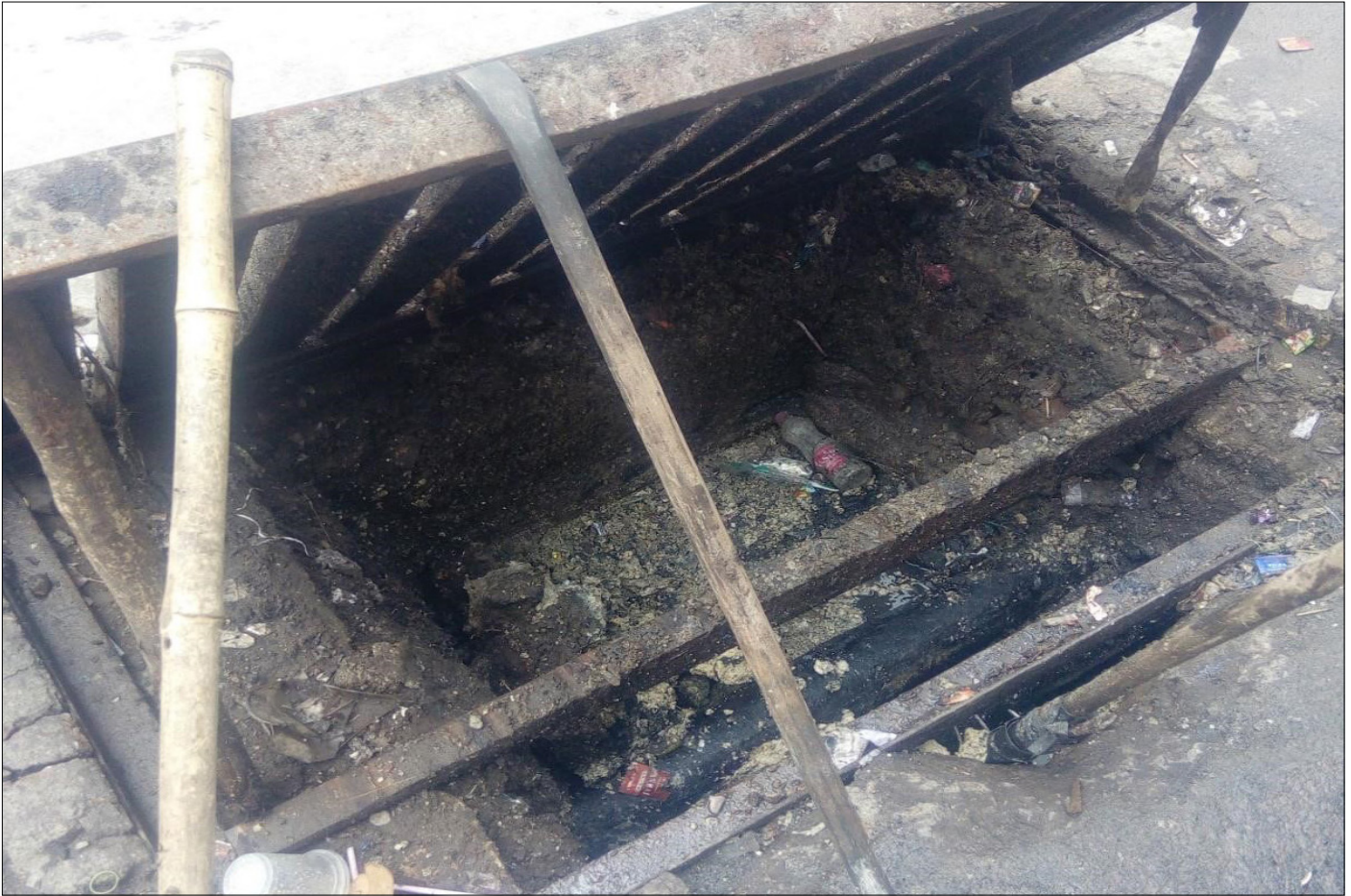
Fig. 14: Choked Sewer Opened for Cleaning
