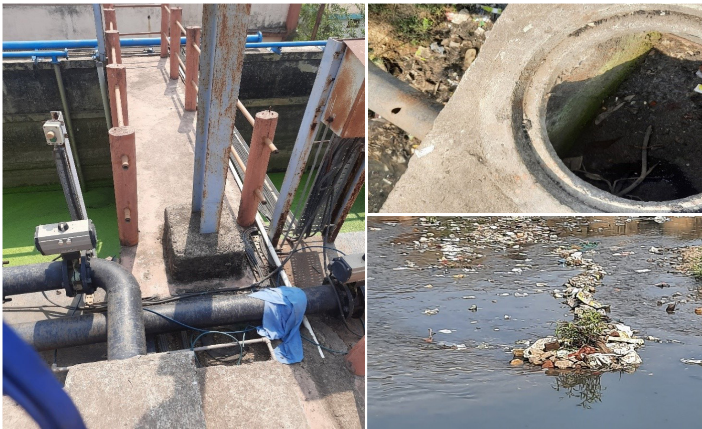
Fig. 10: The Clogged Inlet Chamber, Idle STP with eutrophied water & polluted River in Kawardha
