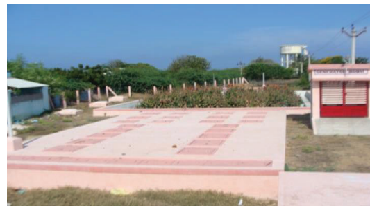
Figure 35: Anaerobic filter at Tsunami rehabilitation housing colony, India
