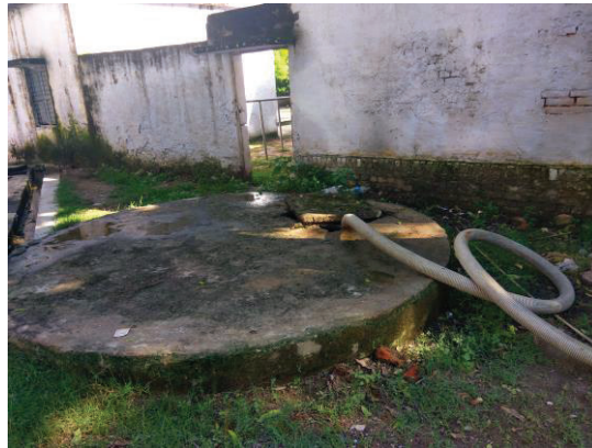
Figure 12: Desludging from a soak pit
