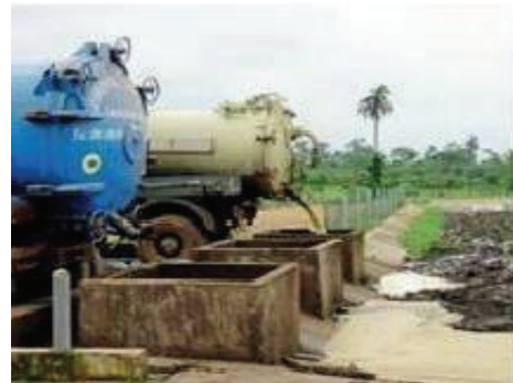
Figure 33: Septic Tanks in Ghana
