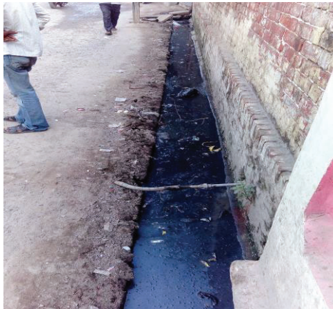
Figure 16: Drains in Unnao
