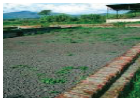
Figure 31: Sludge Drying Beds
