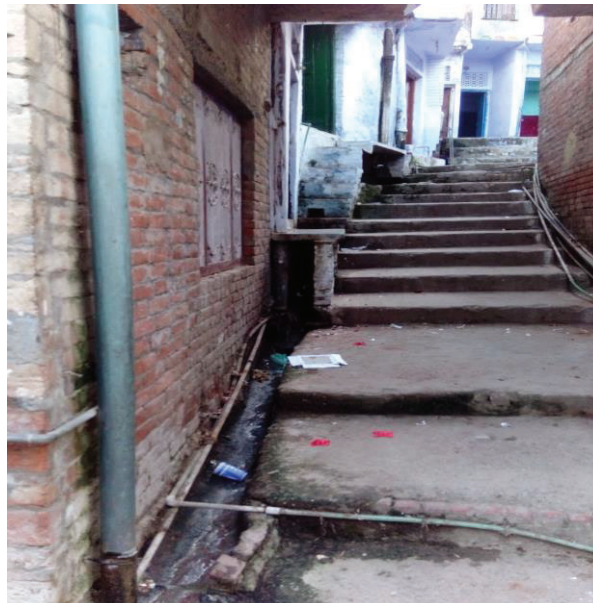
Figure 13: Narrow roads that make access impossible for desludging vehicles
