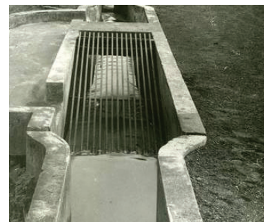
Figure 20: Screening Chamber
