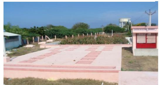
**Supplementary infrastructure and treatment requisite:** If AF is used as a standalone system, then pre-treatment of wastewater in septic tank or ABR is necessary and further treatment of effluent is required for safe disposal or reuse.
