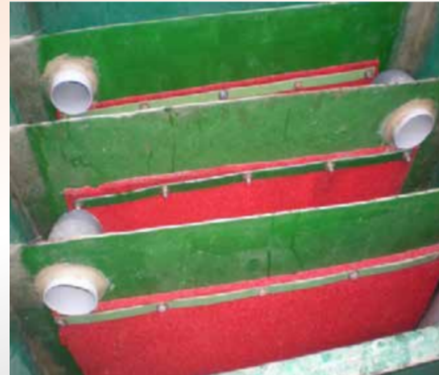
DRDO Biotanks showing different chambers
