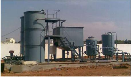
Figure 3: Picture of a MBBR wastewater treatment plant (for representation purpose only; not to the scale)
