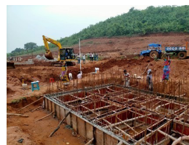
Figure 9: A plant under construction in Odisha
