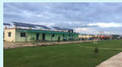
Solar power plant at Bhubaneshwar FSTP
