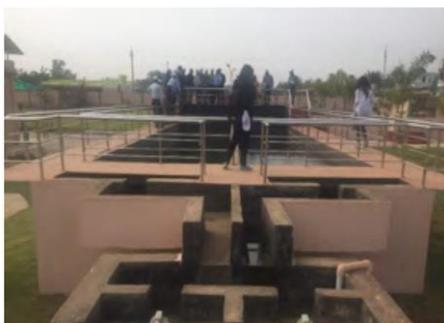
Figure 18 Settling thickening tank, Bhubaneswar (Source: Dhawal Patil, ESF)
