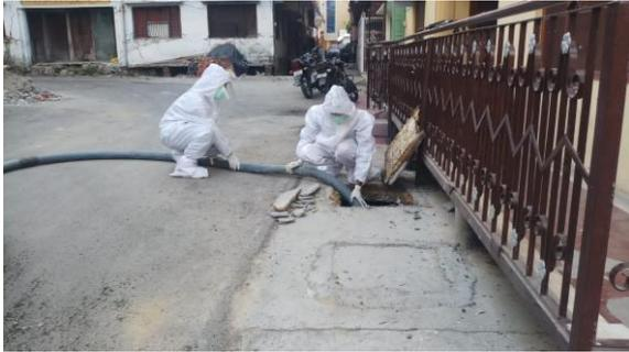
Figure 6 Emptying of Septic tank connected to open drain
