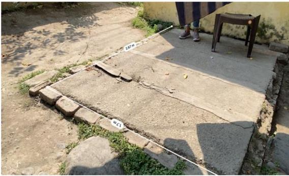
Figure 3 Lined tank with impermeable wall and open bottom (Source: Sachin Sahani/NIUA/2021)
