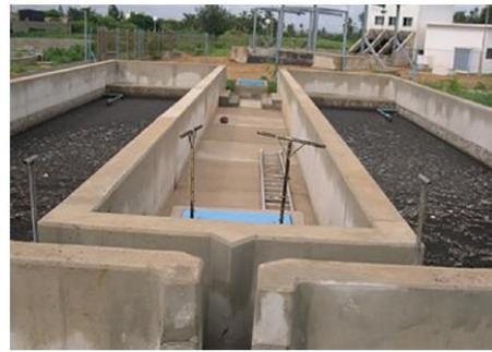
Figure 19 Twin settling-thickening tanks of Rufisque faecal sludge management plant, in Dakar, Senegal ( Source: SANDEC)
