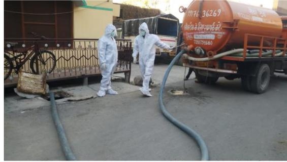
Figure 7 Spillage of Septage during Desludging
