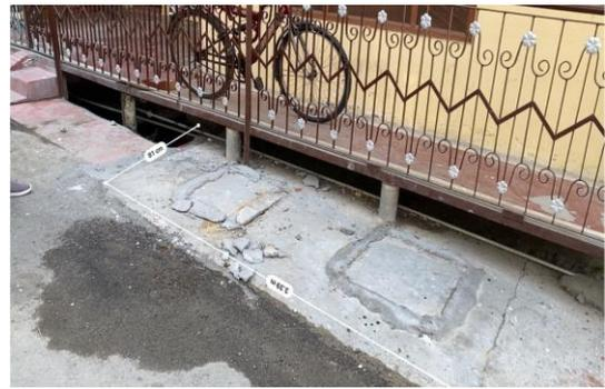
Figure 4 Septic tank connected to Open Drain (Source: Sachin Sahani/NIUA/2022)
