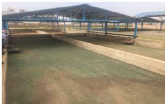
Figure 23 Unplanted sludge-drying beds, Bhubaneswar
