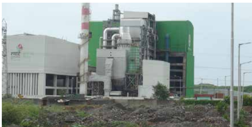
Figure 20 Waste to Energy Incineration Plant in Kathonda
