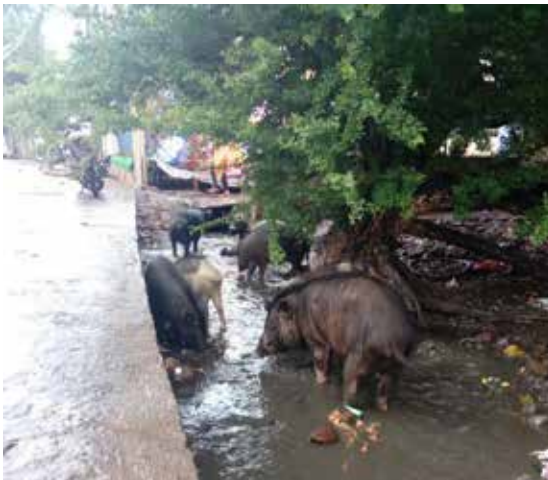
Figure 6. Open drain with Pigs feeding in Gupteshwar Area
