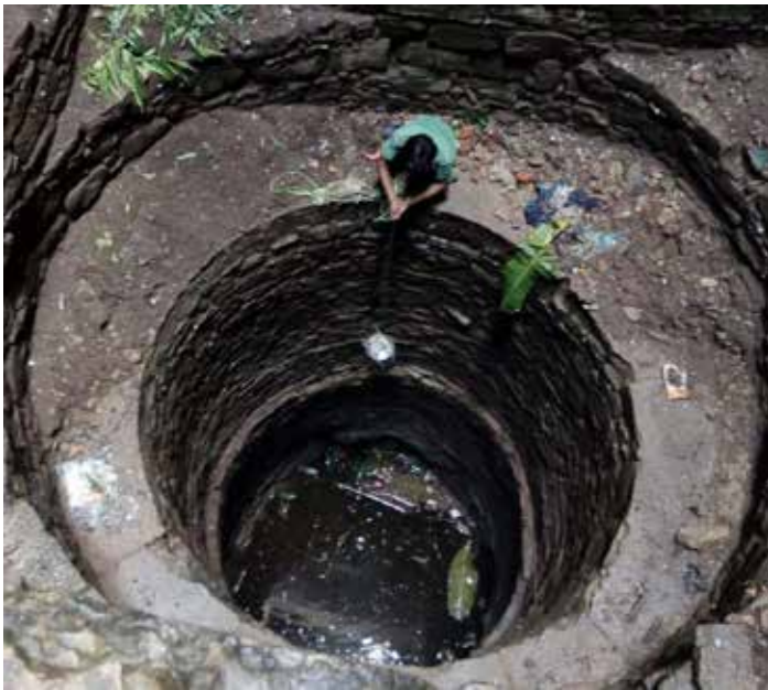
Figure 6: Open Well in the Fort
