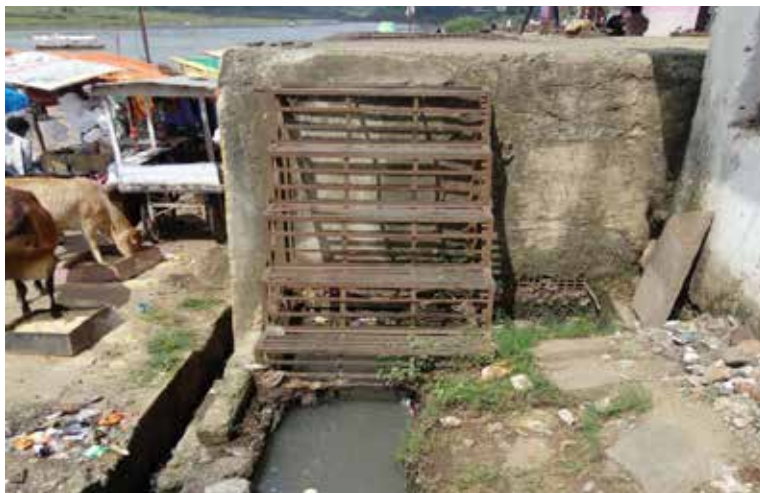
Figure 19 : Open Drain near Gwari Ghat on the Narmada River
