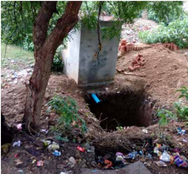
Figure 2. Single Pit Latrine in Malviya Ward
