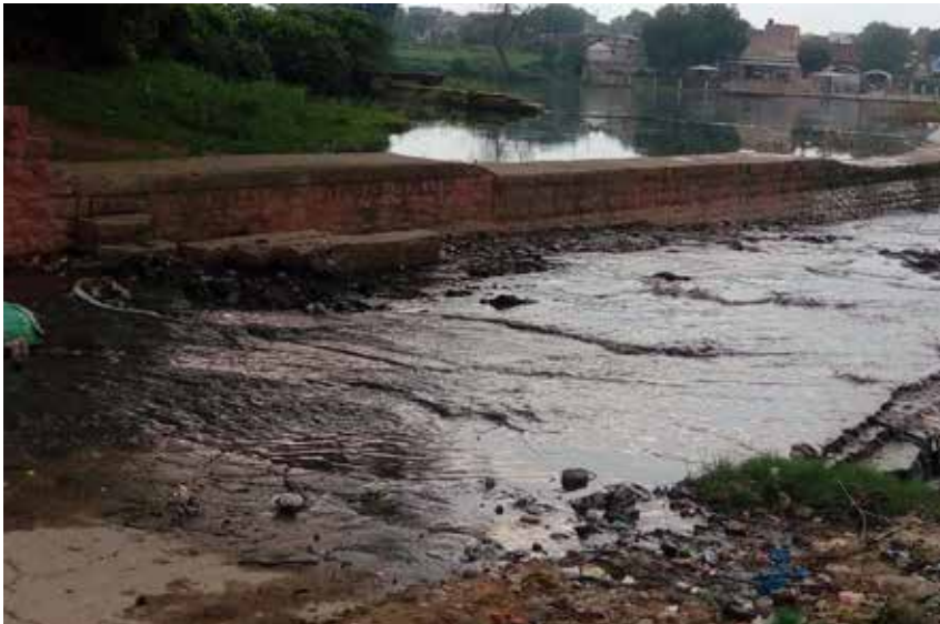
Figure 9. Nala emptying into Seep River below Banjara Barrage
