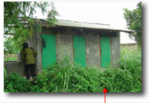
Abandoned Public Toilet
