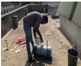
Leak Detection if any
